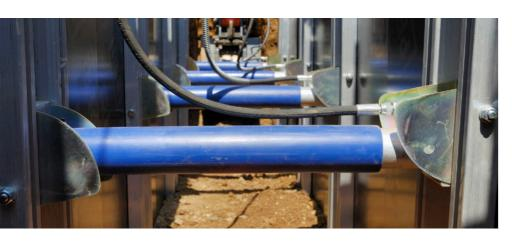
The Quick Shore 260 series is specifically intended for shoring depths of up to 2.00 m.
